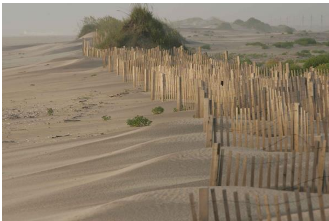
Figure 4. Example of sand fences used in coastal region
