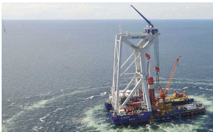
Figure 8: Big Bubble system to reduce underwater noise from pile-driving operations during the construction of an OWF [29]
