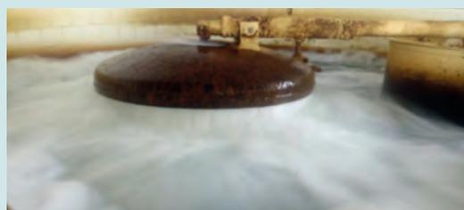
Figure 176 - Water pressure dissipation using a load breaker
