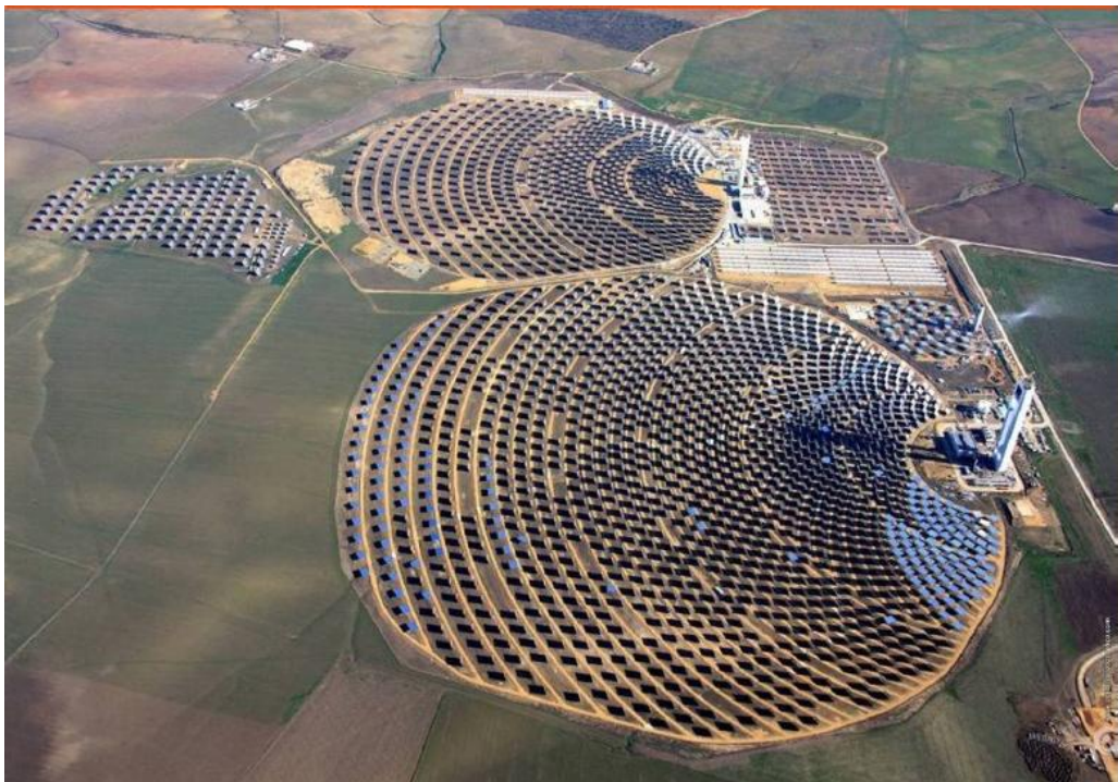
Figure 7 – Solar plants PS 10 and PS 20 in Sevilla (Spain)
