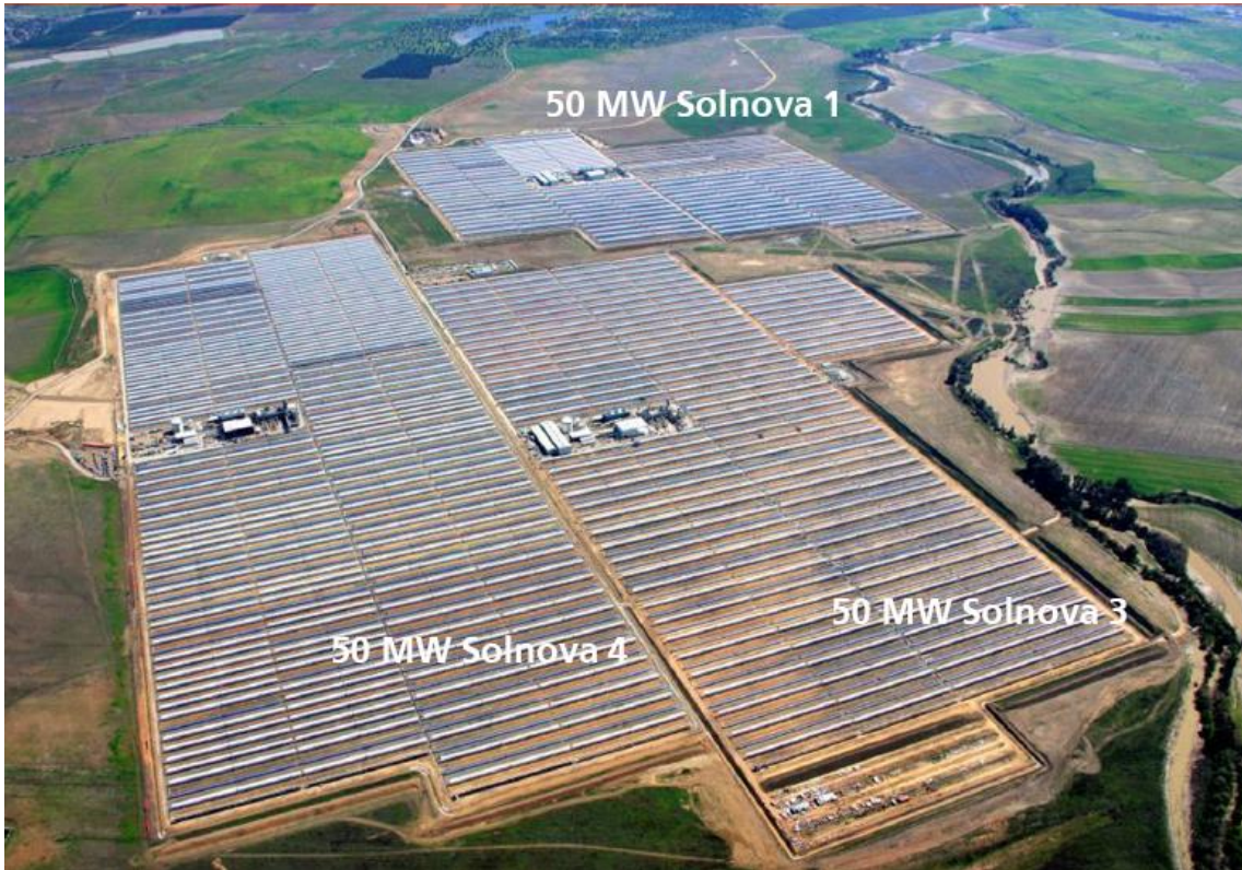
Figure 8 – Solar plant in Solnova (Spain)
