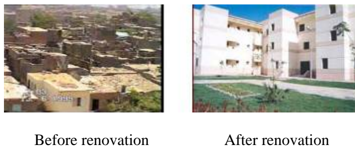
Figure 11: Zeinhum informal housing settlement before and after renovation, (17).
