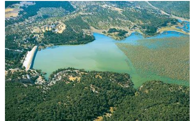
Nebeur Dam in Tunisia (Source: Econostrum)
